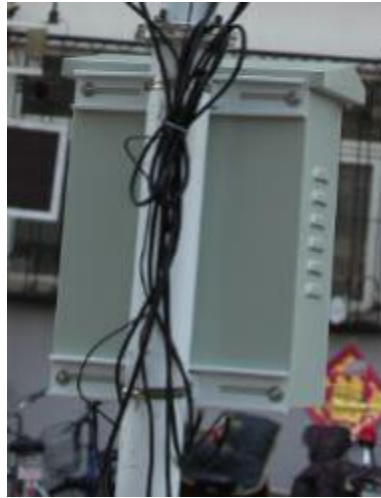
Installation completed rear view
