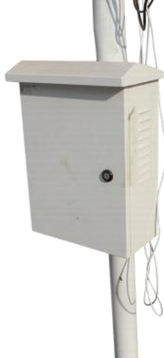
Installation completed front view:
